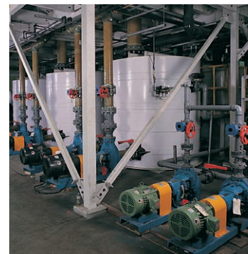
Multi-stage external recirculation system.
