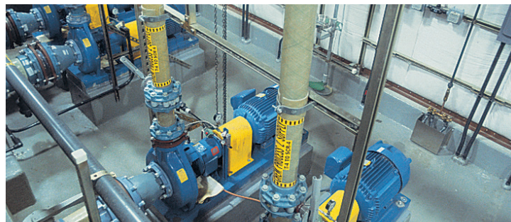
Dual pump back-up on multi-stage system. ANSI design.
