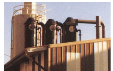
Tri-NO x scrubber through-the-roof installation.
