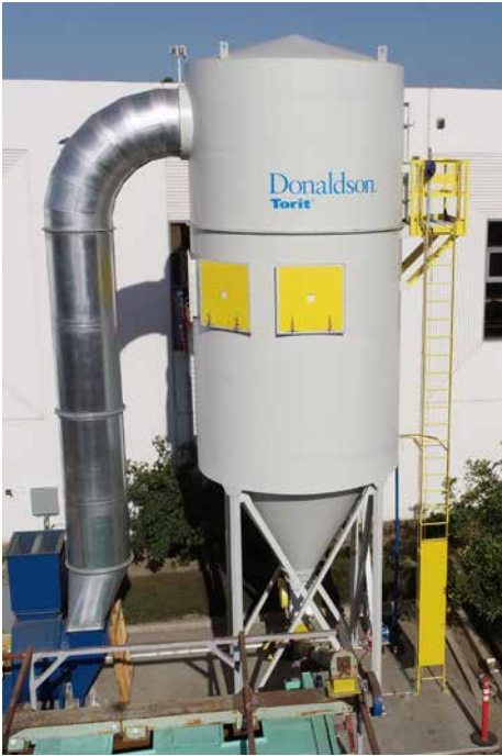
200RP at Skateboard Manufacturing Facility
