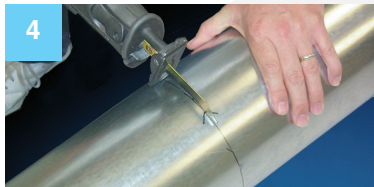
Drill access hole, then cut Pipe with saw.
