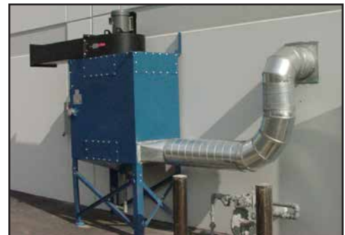
A) Outdoor installation of a Donaldson® Torit® Dryflo® DMC-D2 mist collector using spiral ducting
