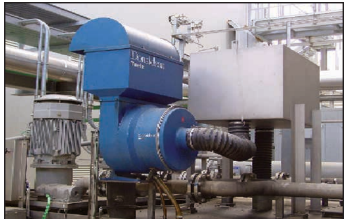
AF) Example of a weather hood over the exhaust of the centrifugal mist collector to avoid intake of rain, debris, etc.
