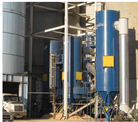
RF - Grain Terminal 34,000 cfm (57,754 m 3 /h)
