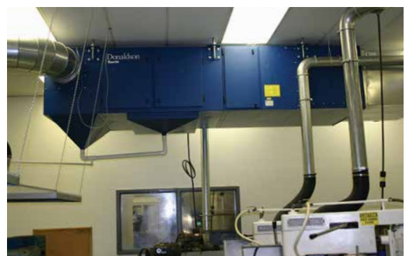
Modular Mediafilter™ on Grinding 2,000 cfm (3,397 m 3 /h)
