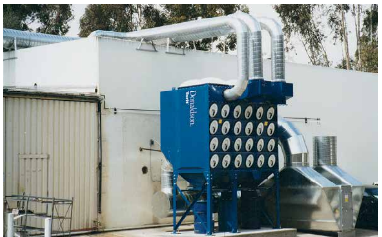
DFO on Metal Grinding 31,000 cfm (52,658 m 3 /h)
