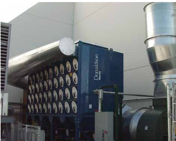
DWS on Custom Hand Grinding 38,500 cfm (65,398 m³/h)
