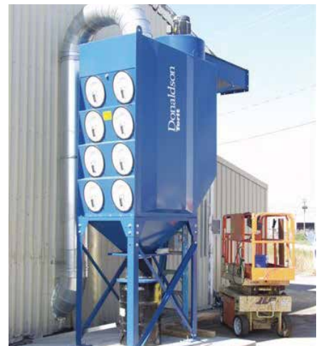
DFO on Plasma Cutting 5,000 cfm (8,493 m³/h)
