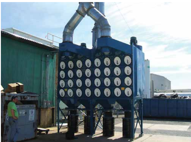
DFO on Thermal Spray 8,500 cfm (14,439 m 3 /h)
