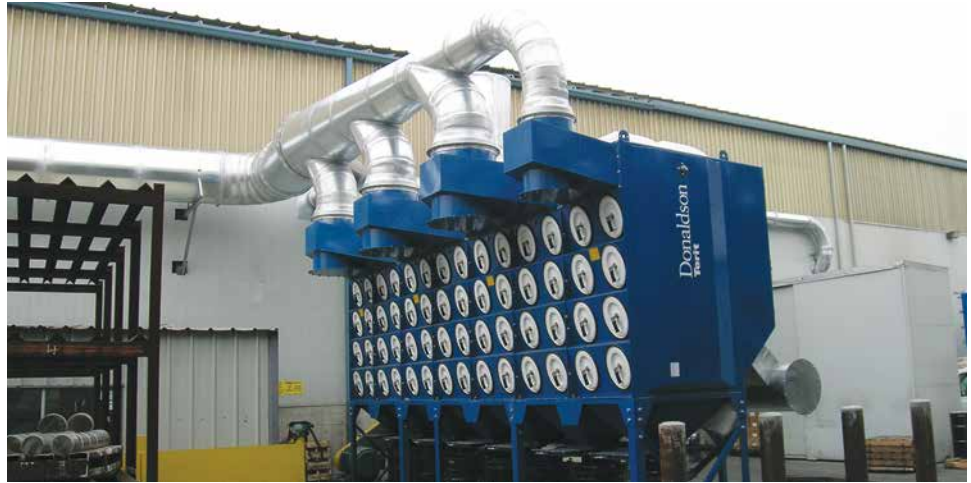
DFO on Grinding 74,000 cfm (125,700 m³/h)
