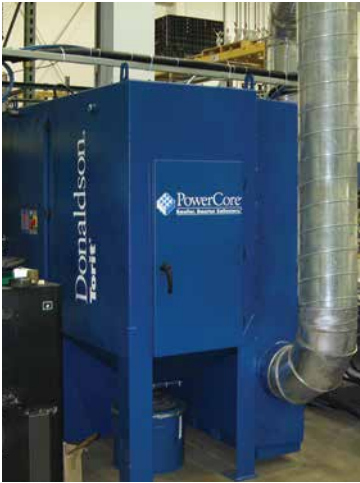
TG on Plasma Cutting 2,300 cfm (3,90 m³/h)
