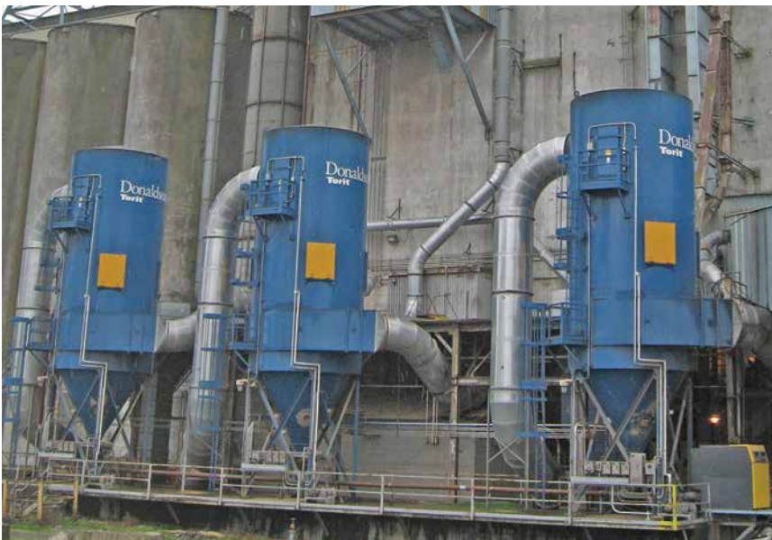
RF - Grain Terminal 61,000 cfm (103,618 m 3 /h)
