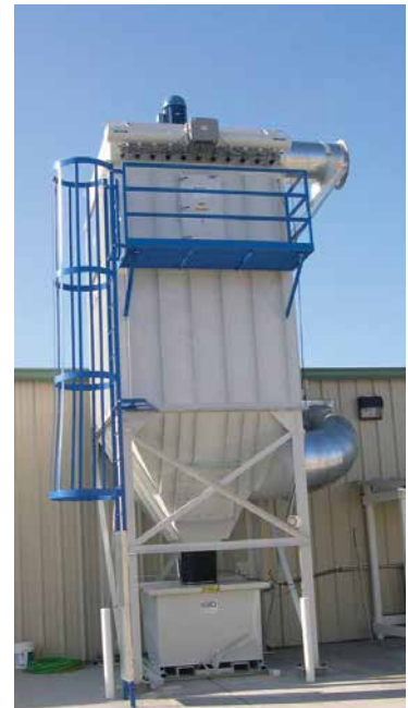
FS on Woodworking 20,000 cfm (33,973 m 3 /h)
