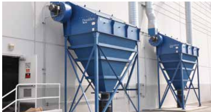
CPC-24 - Paper tissue manufacturing 7,600 cfm (12,910 m 3 /h)
