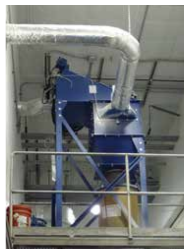
CPC-3 - Powdered milk dust in cheese factory 1,200 cfm (2,038 m 3 /h)
