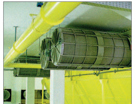
Explosion protection at milling hopper in breweries
