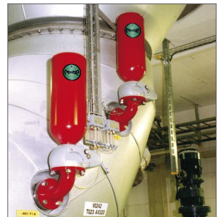
Q-Bic in a large pipe
