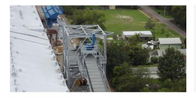
Placed at transition points or at the head and tail section of enclosed conveyors, 4 PowerCore® CPV collectors avoid the need for costly ducts as well as the need for material handling equipment to move collected dust to storage.
