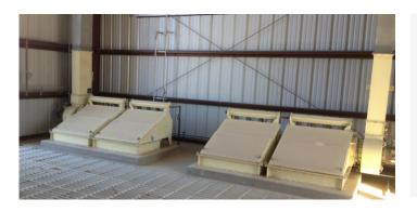
For new or replacement dump pits, 3 PowerCore® CPV collectors require smaller, quieter fans that reduce noise exposure and lower costs.
