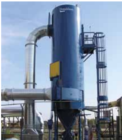
RF DUST COLLECTOR
