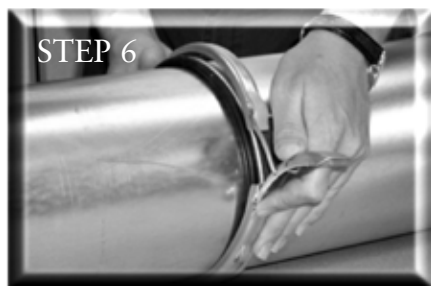
Snap clamp over O-ring and one end of nipple.
