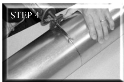
Drill access hole then cut with saw
